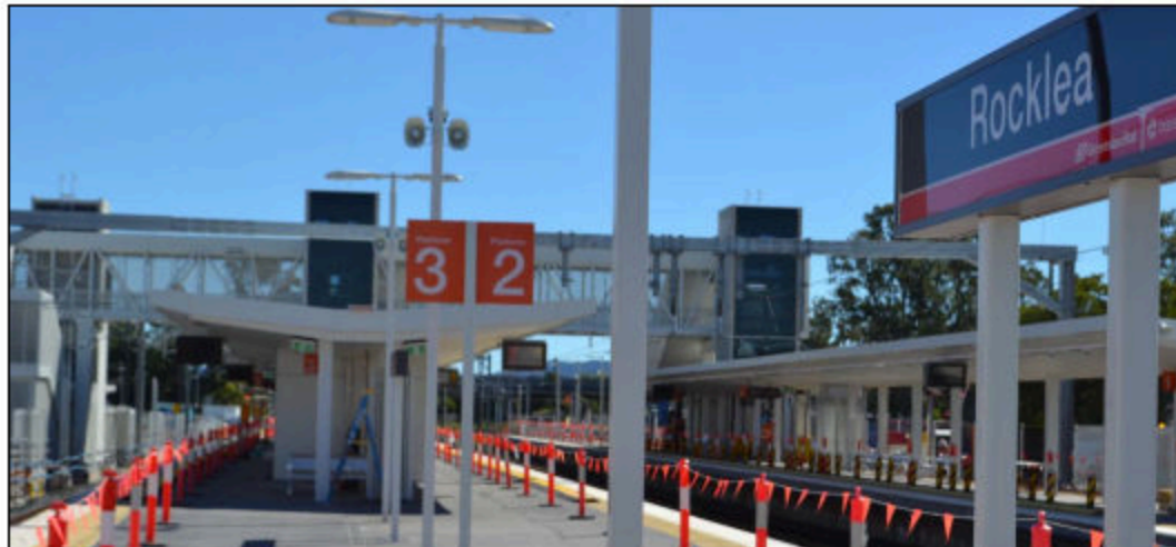
Rocklea station platforms 2 and 3.
